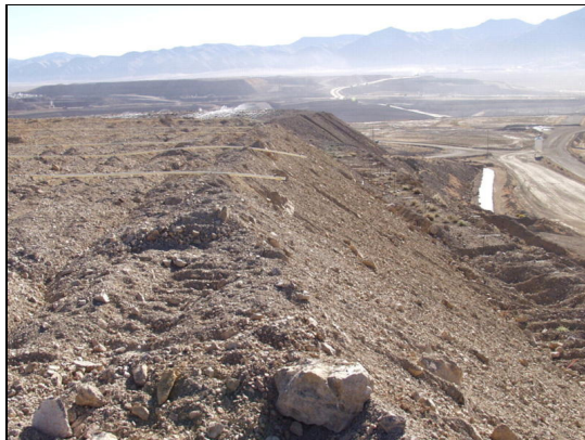
Figure: 4 Gold Acres heap leach pad showing side slopes of the test region. The plastic pipes visible were used to supply the leach solution via drip and spray irrigators
