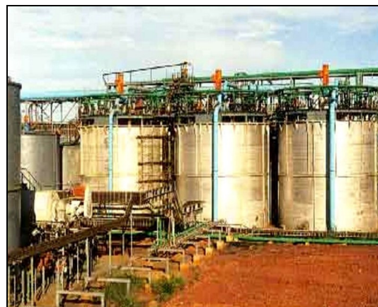
Figure: 7 Bioleaching tanks
