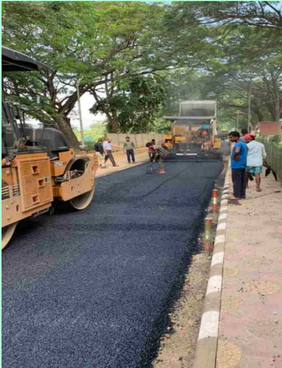
Fig. i): Plastic tar used in Erode road, Tamil Nadu
