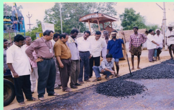
Fig. iii): Plastic tar used in Madurai Kombadi road
